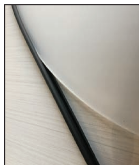
Lens Gasket required for IP66 Rating
